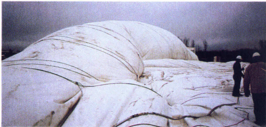
Bubble being inflated and heated simultaneously by BABFAR Equipment.
